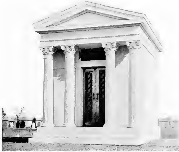
Number 8909. Classic structure in the Greek Corinthian style. The grille work of the bronze doors is backed by glass shutters, permitting a view of the interior, which is finished in light veined Italian marble, and contains eight receptacles. Erected for Mrs. Harriet Gould Jefferies, in City Cemetery, Augusta, Ga.
